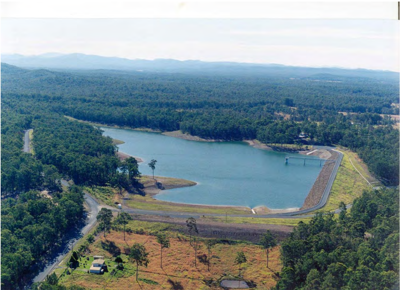
Steuart McIntyre Dam completed in 2001 has a capacity of 2,500 Megalitres
