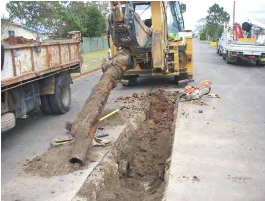
Replacing old water pipe
