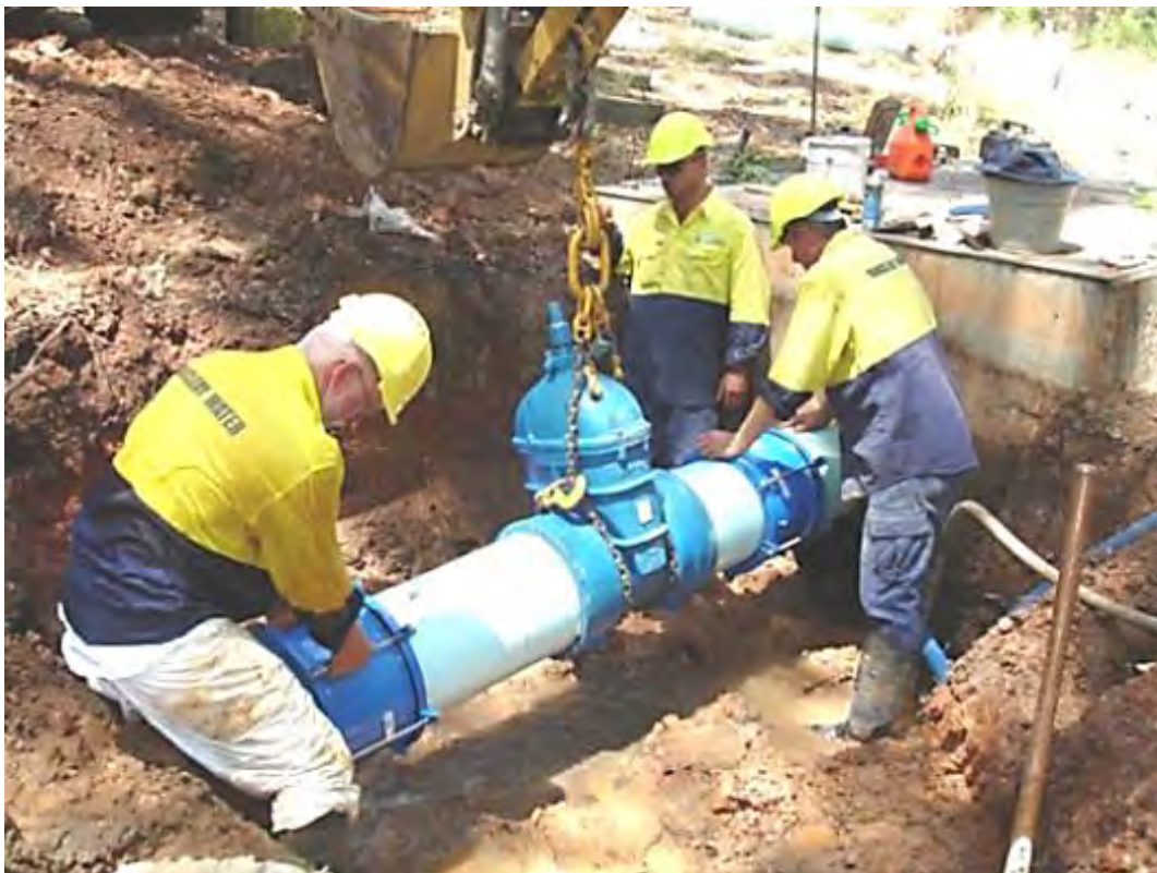
Replacing a valve at Potters Hill Reservoir
