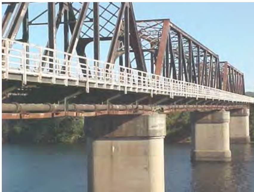
Asbestos cement main to be removed from Kempsey Railway Bridge
