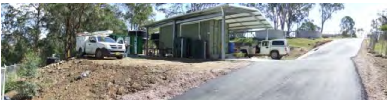
New Bellbrook Treatment Plant constructed in 2010
