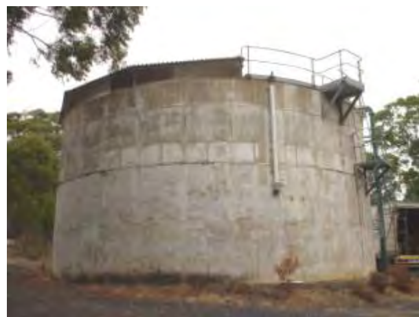
Hat Head concrete reservoir
