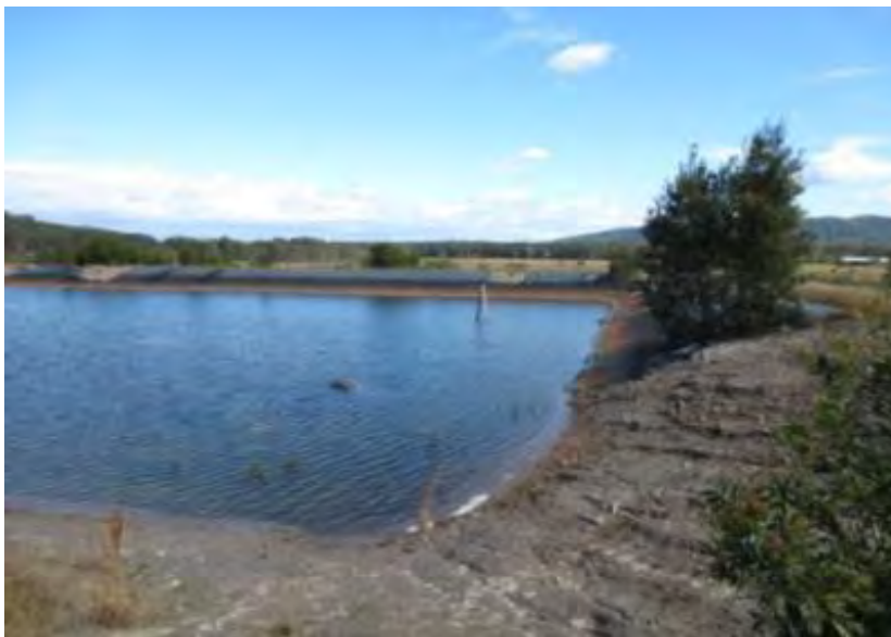
Hypalon Dam at Crescent Head Water Treatment Plant
