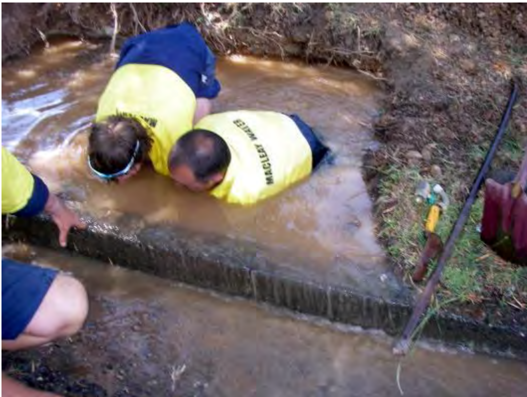
Repairing a broken water main
