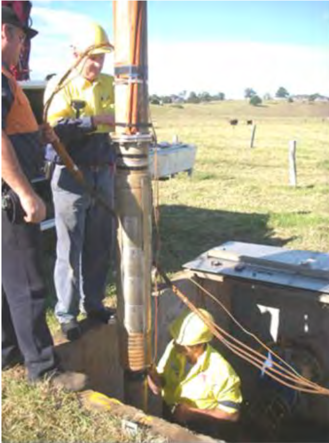
Replacing a bore at Sherwood
