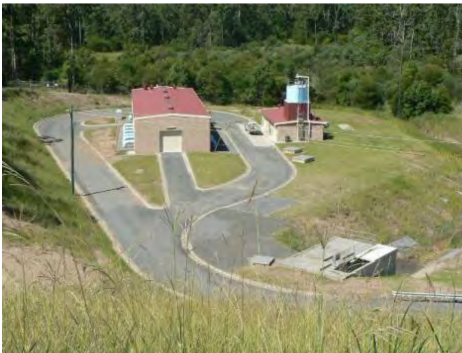
Pump station & dosing station at Steuart McIntyre Dam A new water treatment plant is planned for 2026/27
