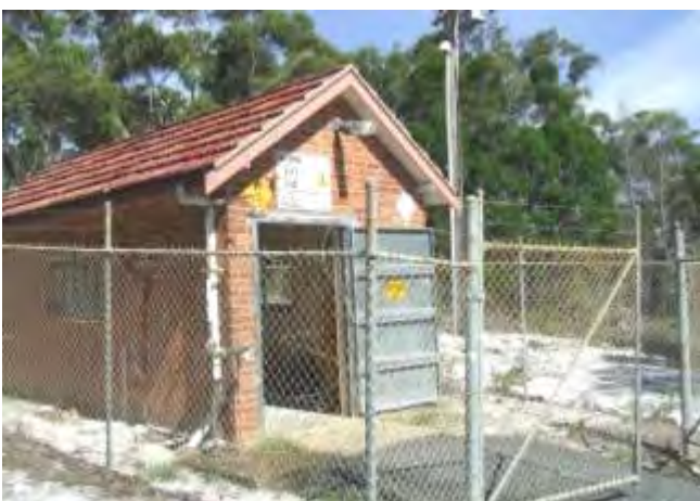
Dosing station at Hat Head
