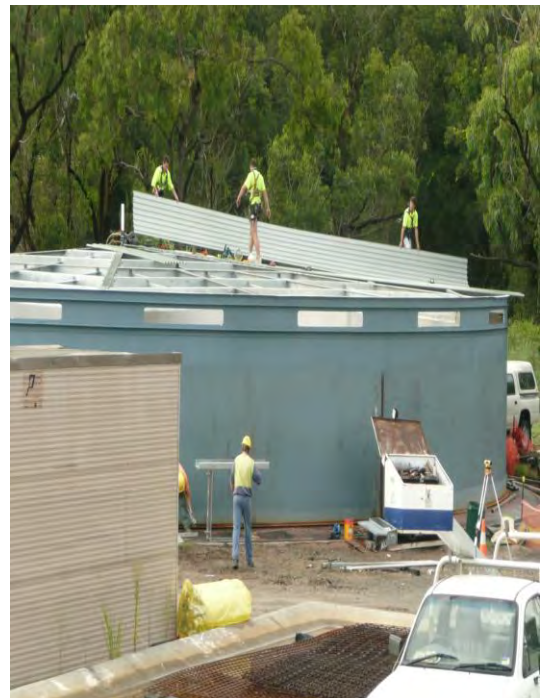
A one megalitre above ground balance tank was constructed at the new recycle water treatment plant at South West Rocks for storage of tertiary treated effluent prior to use at the recycle water treatment plant
