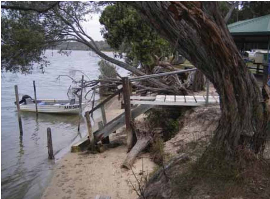
Figure 9 Image showing wave induced erosion
