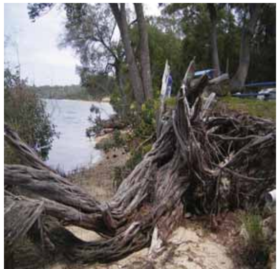
Figure 6 Steep bank erosion
