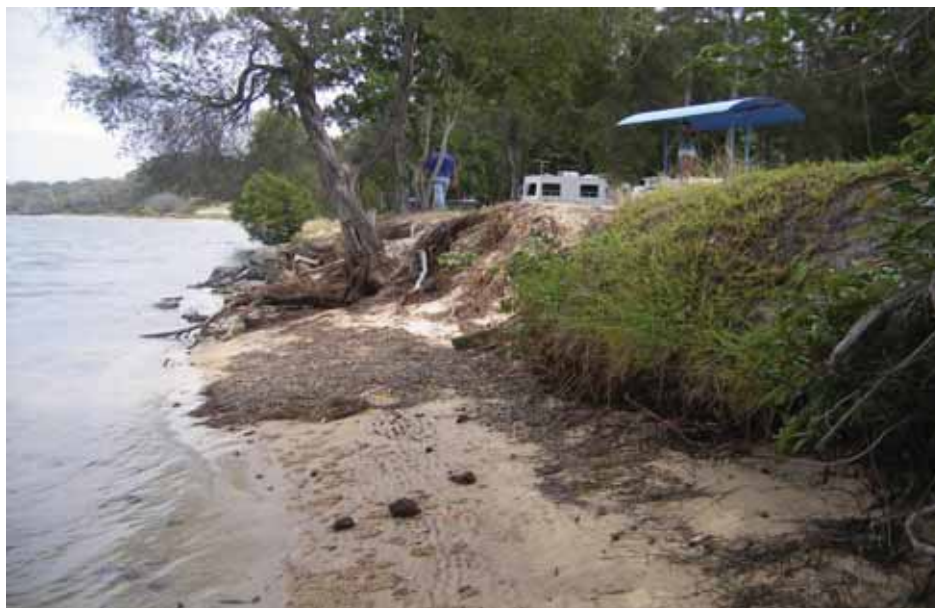
Figure 8 Image showing toe scour erosion along foreshore
