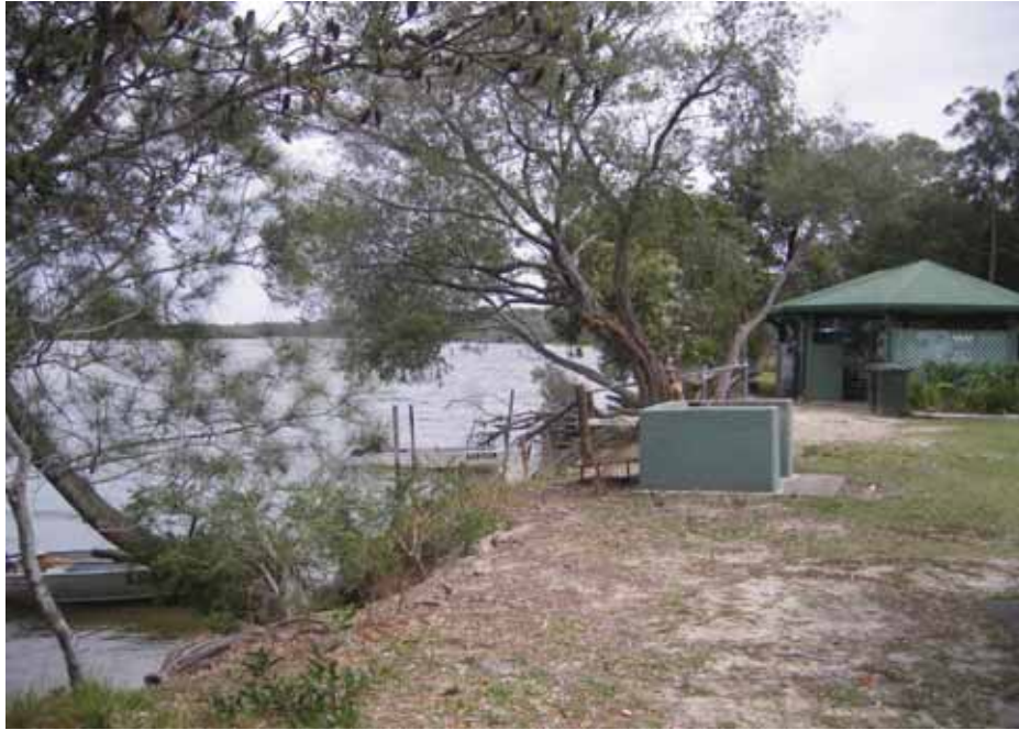
Figure 4 Public infrastructure under threat from bank erosion
