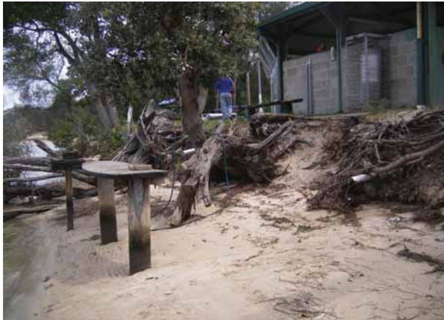
Figure 7 Showing surface scour resulting from pedestrian movement down the bank
