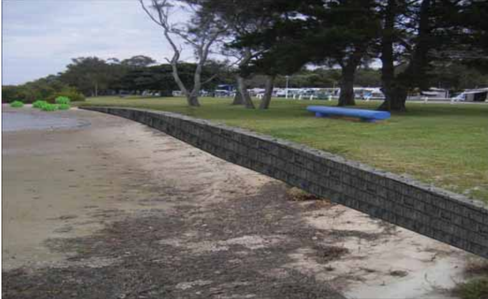
Figure 13. Proposed erosion remediation work – Zone 1
