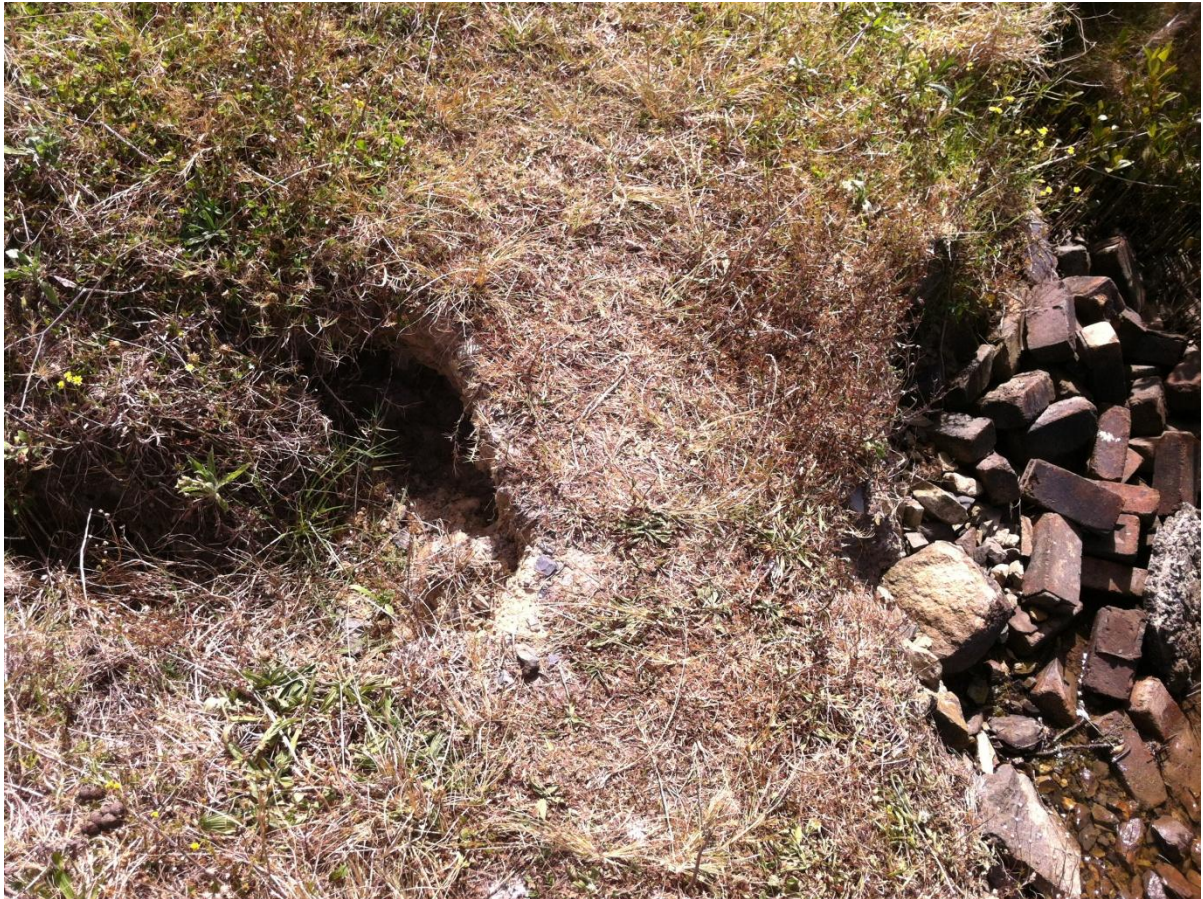
Figure 29 Collapsed tunnels on Teal Lagoon berm, caused by sub surface erosion of the soil overburden
