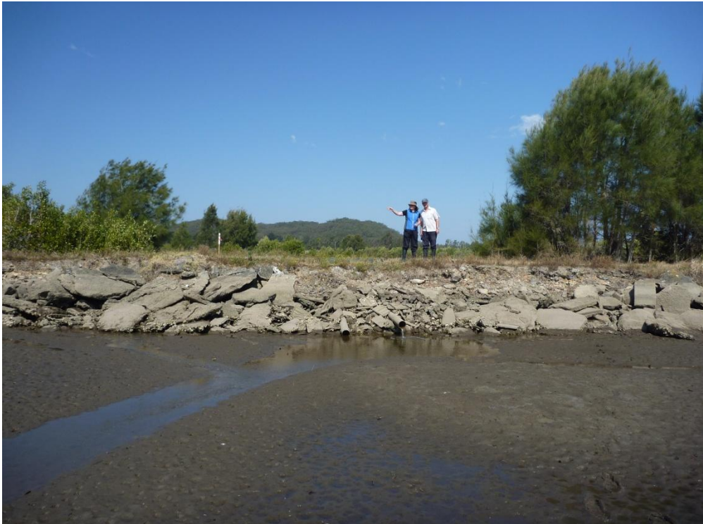
Figure 28 Water discharging through pipes and berm during low tide conditions
