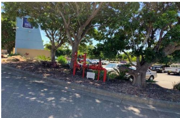
Photo 11 – Attack Hydrant to be relocated
