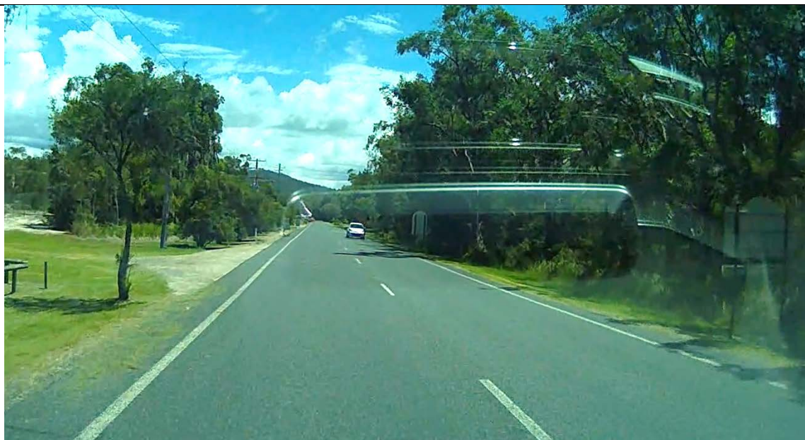
Figure 2.3: Pacific Street, looking west towards Crescent Head Road
