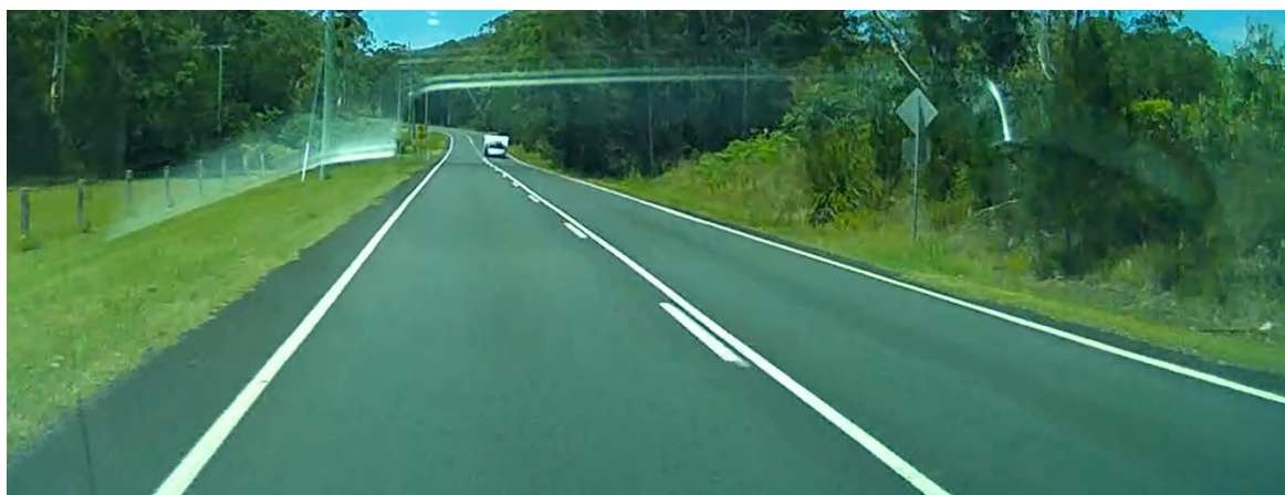
Figure 2.4: Crescent Head Road, showing a recently upgraded section of road
