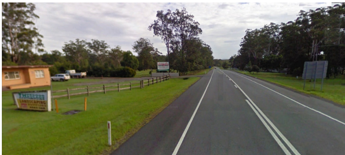
Figure 5.1: Northbound view of Thurgate Haulage access from Macleay Valley Way
